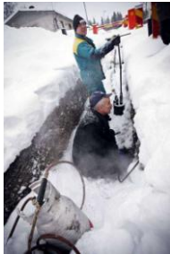
Freezing protection of water pipes
